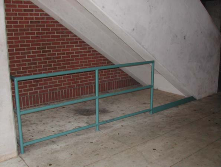
Fig 3. Area under stairs, with blocking rails
